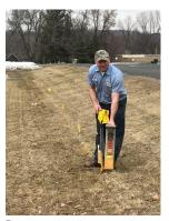
When a request to locate is called into Diggers Hotline, we use a device like this to locate our pipelines... so an excavator doesn't get a surprise.
