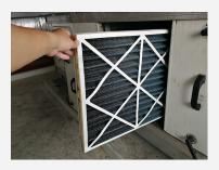
One of the easiest ways to prevent wear and tear on your system is to check your air filter. These filters help your furnace and air conditioner remain energy-efficient and improve your home's air quality. This is one type of maintenance that you can handle by yourself. If the filter has a large collection of dust or dirt, you will want to replace it with a clean filter.
